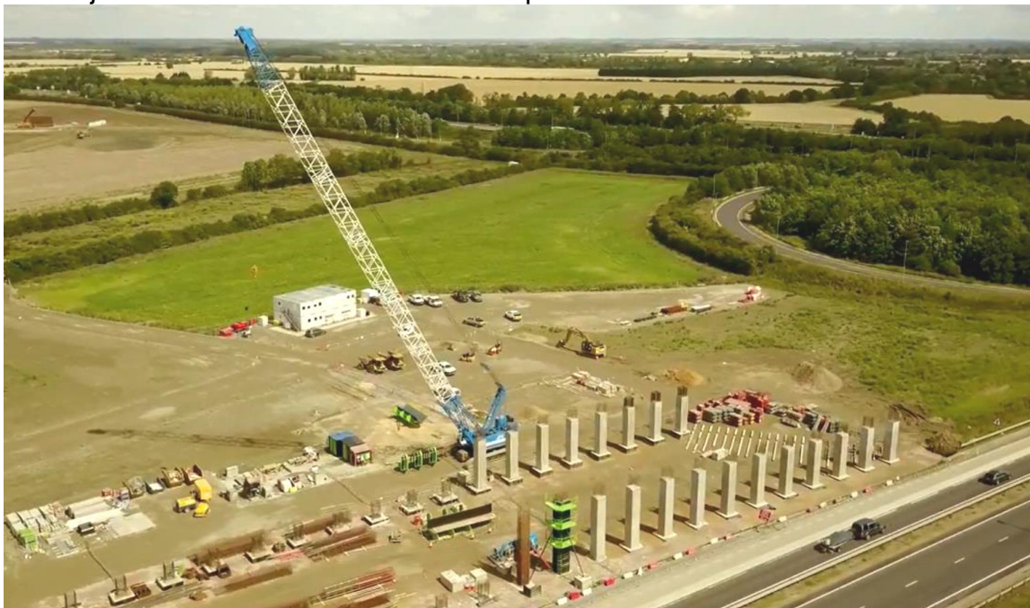
Bridge columns under construction next to A428.
